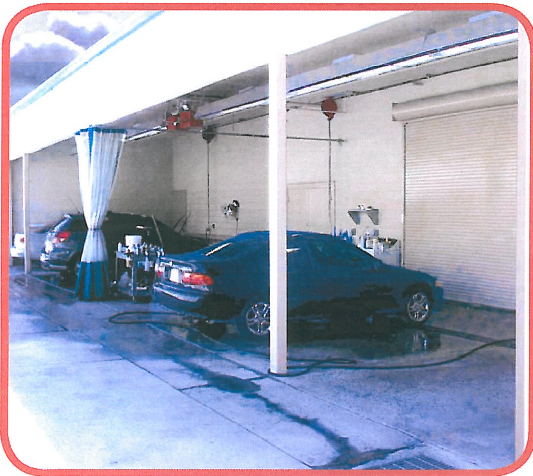
Covered car wash – drains to clarifier
